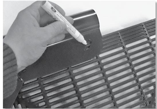
5. Remove the AeroFlap® from the bracket, place on a solid surface and use a drill to make the necessary holes.
